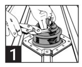
Trim the cone to suit pipe size using sharp tin snips.
